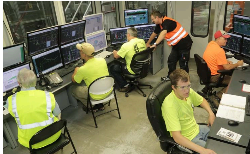
▲ Operators in the control room for TM1 and TM2.
